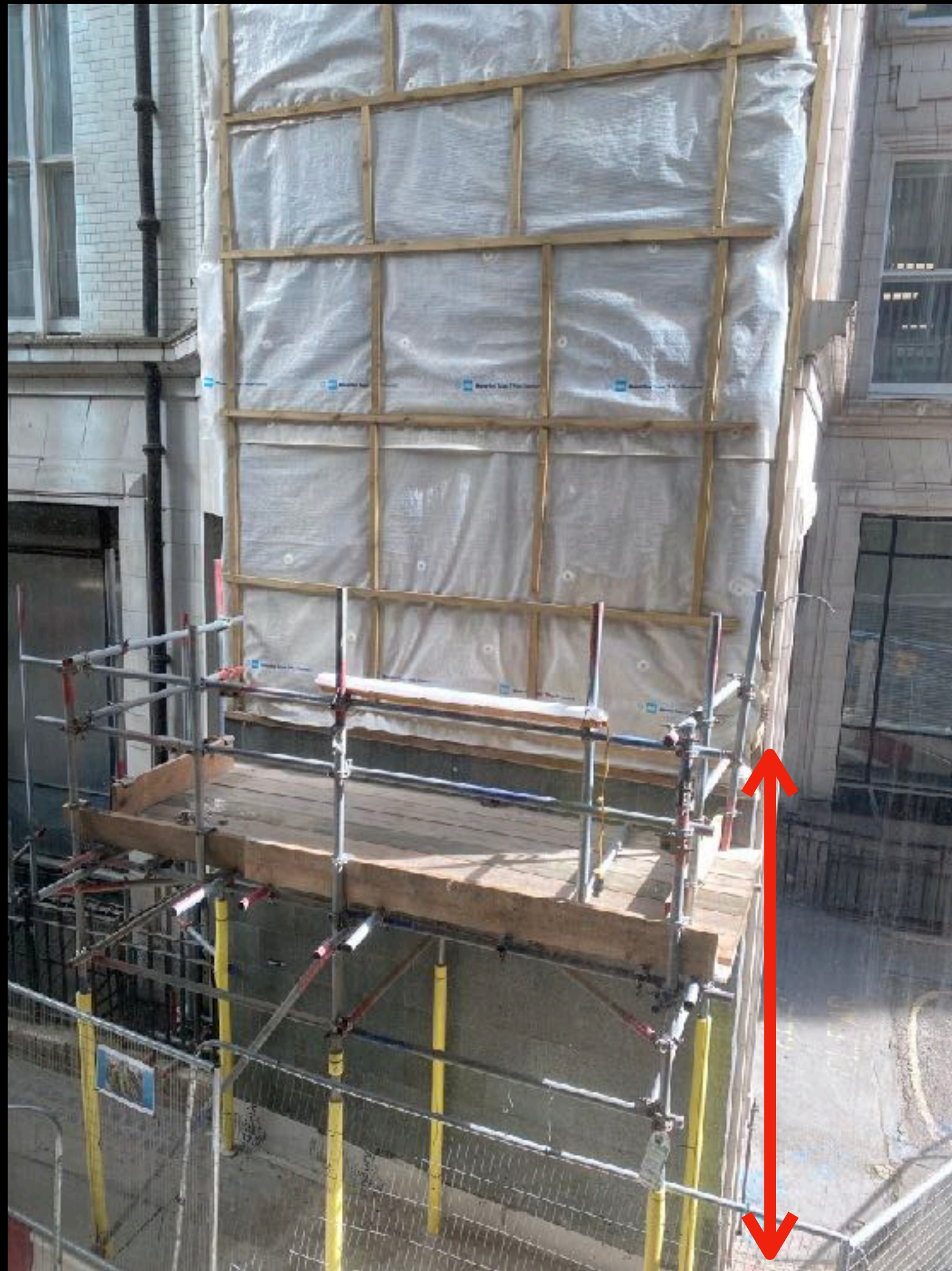
Artwork begins 3.5m above ground level.
